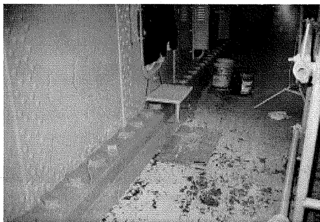
Section of deck that has been scraped and primed
