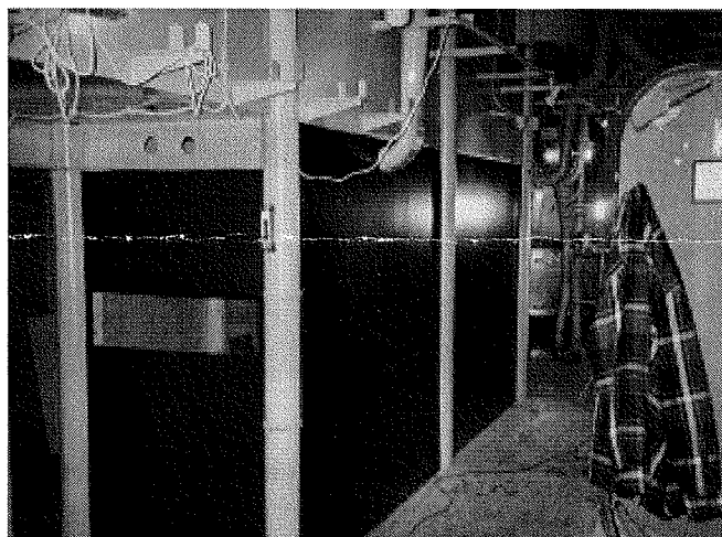
Section of deck that has been scraped and primed
