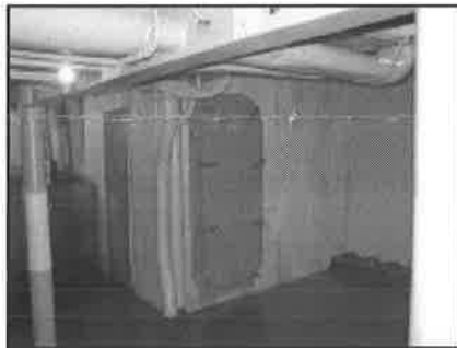
Exterior of radar room before porthole was installed and painting done.
