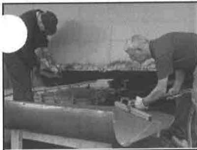
John Hemminger grinding duct section and Jack Floyd cutting steel plate.
