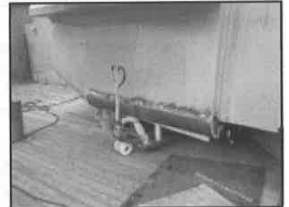
Plate lifted into place.
