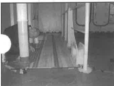
John Hemminger taping joints in wood deck.
