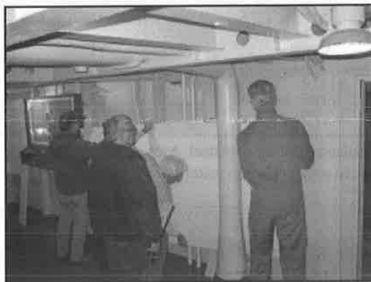
Sliding plywood sheeting in place
