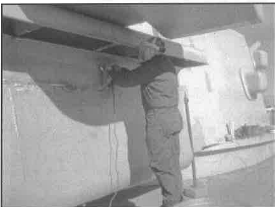
John grinding welds.
