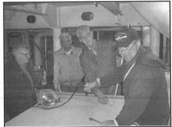
Jack, Al, Jim and Roland cutting plywood.
