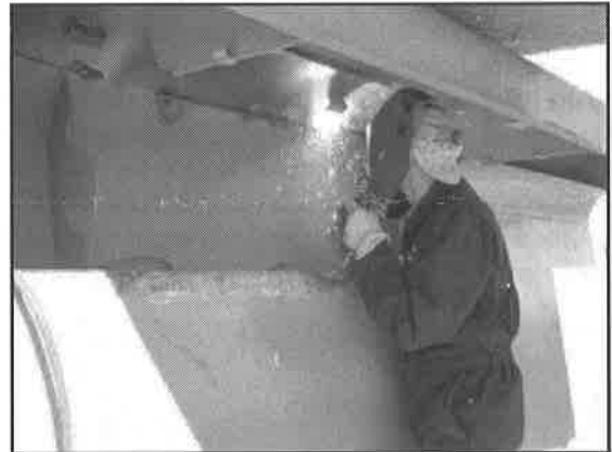
Harry welding new steel plate in place.
