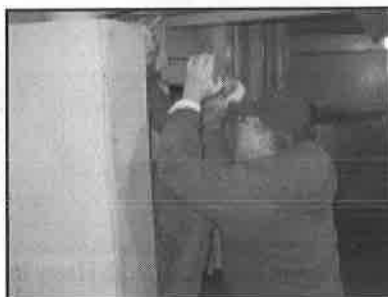
Roland using nail gun to attach front panel.
