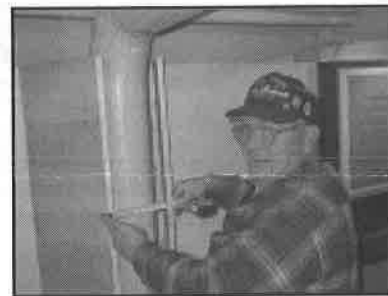
Henry checking measurements before cutting front panel.
