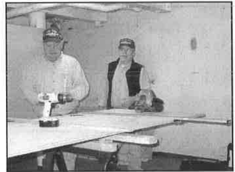
Henry MacKay and Roland Cote cutting plywood.
