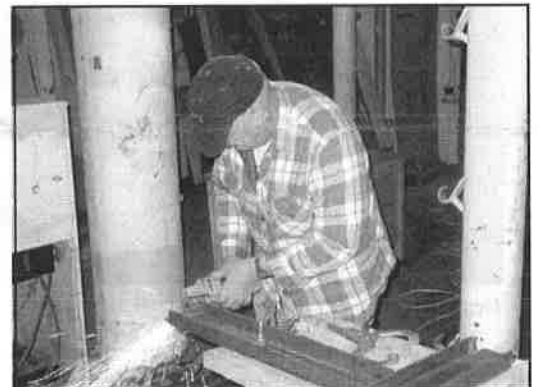
John Hemminger grinding channel iron for the platform
