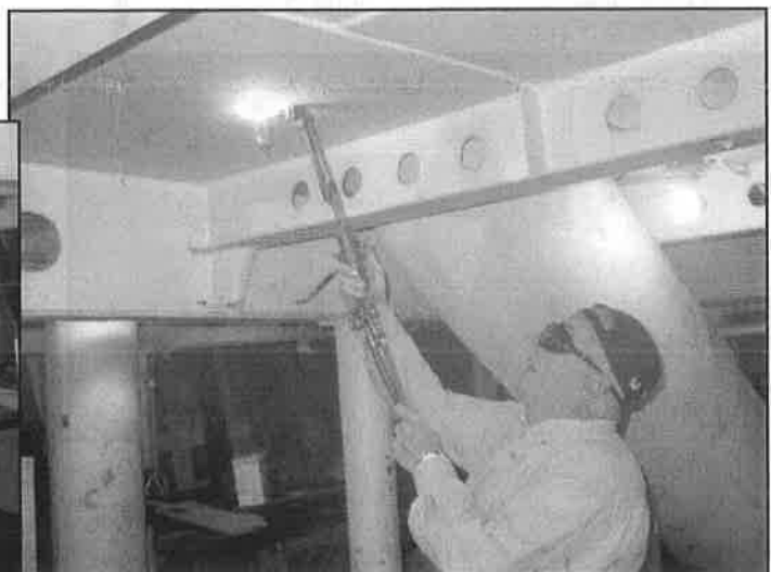
Henry (above) cutting brackets off the overhead.
