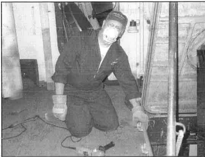
John (left) and Roland (below) grinding welds flush with the deck. Both are very proficient as they had plenty of practice from working on the YAGR'S exhibit.
