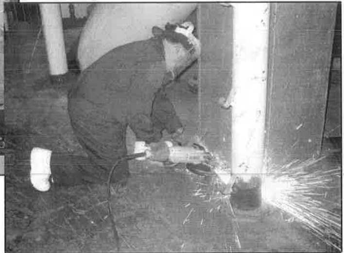
John (left) and Roland (below) grinding welds flush with the deck. Both are very proficient as they had plenty of practice from working on the YAGR'S exhibit.
