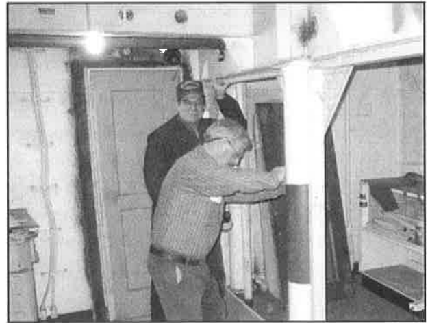
Tom and Jack installing a section of framing
