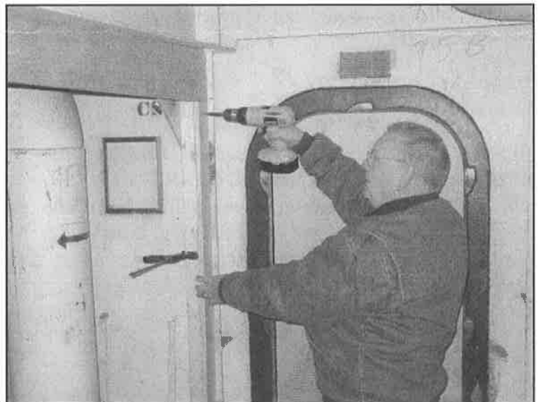
John installing side trim
