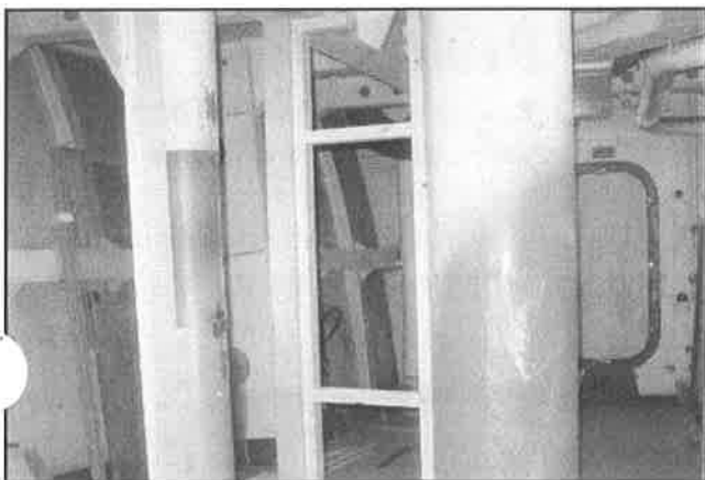
New bulkhead framing
