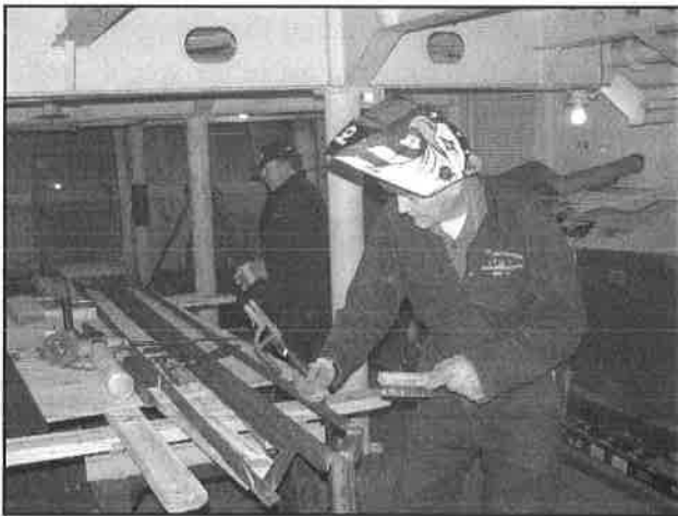
Harry welding stringers
