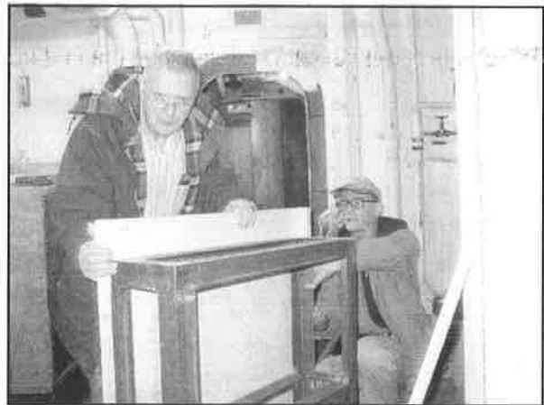
John and Dave working on a side panel.
